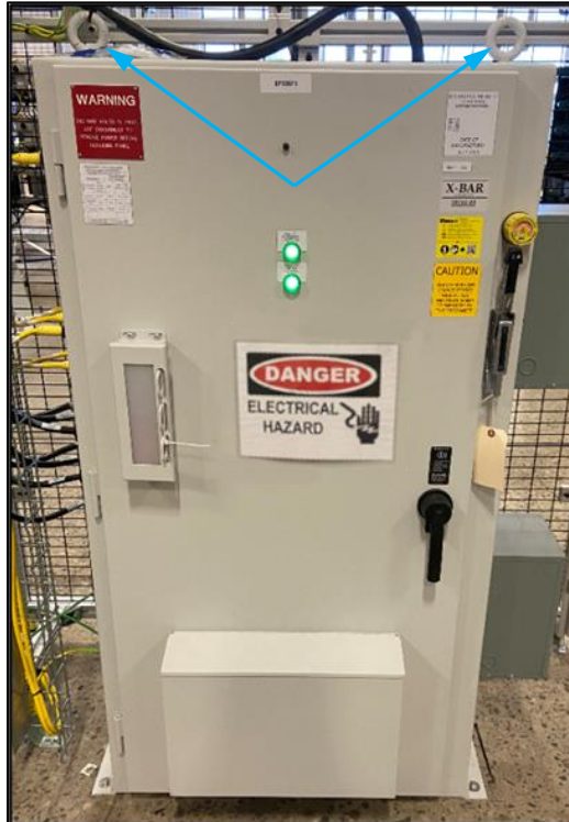
Figure 8-1. PDP Lifting Points.
