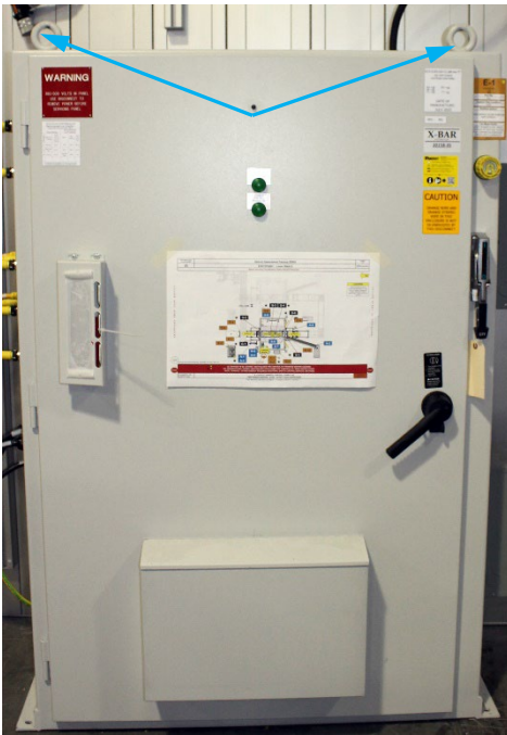
Figure 8-2. PDP lifting points.
